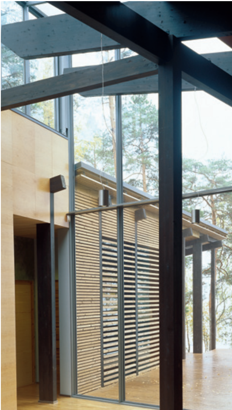
Built for exhibition purposes by Finnforest, this summer cabin is based on building technics.
