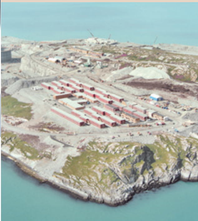
A large order of temporary barracks was supplied by Moelven Modular Buildings for the Snøhvit gas field project at Melkøya, outside of Hammerfest, Norway.
