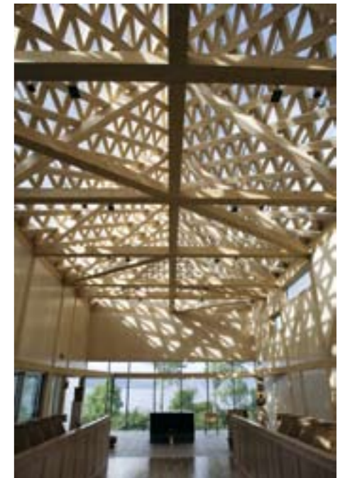
Moelven Limtre AS has supplied the spectacular glulam structures used in the Maria convent in Nord-Trøndelag. Moelven Limtre AS is Norway's leading supplier of standard and customised glulam structures for Building projects.
