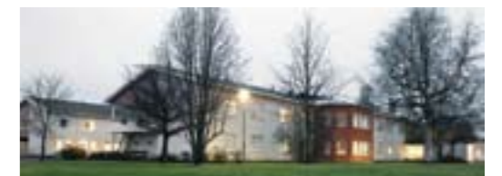
Moelven Årjäng Säg AB supplies distance heating to Årjäng municipality via its distance heating facility at the sawmill. Bioenergy is an important emerging market segment for Moelven, and the Kvarnåsen Retirement Home is an example of an institution heated with energy generated from ecological chippings and bark from the plant. Moelven has initiated heavy investments in the development of the bioenergy sector as a new business opportunity.
