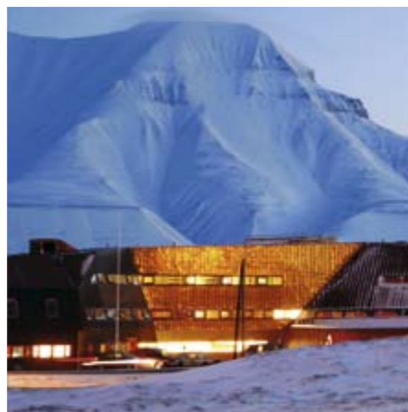
Moelven Limtre AS supplied glulam structures to the new Svalbard research park in Longyearbyen
