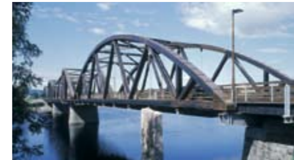
Sawn wood from Timber is used as a component product in the production of glulam. The photo shows the glulam structures used to build the Flisa bridge crossing the river Glomma.
