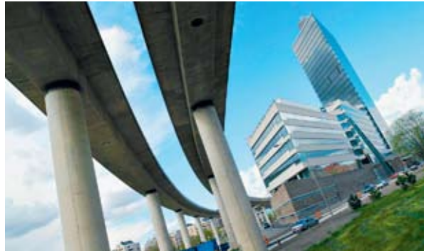
The Kista Science Tower, northwest in Stockholm, consists of six buildings with business offices, conference and exhibition facilities. The tallest building has 32 floors. Moelven Eurowand AB has delivered system walls for the complex. Total office space at the Kista Science Tower is approx. 43 000 square metres.
