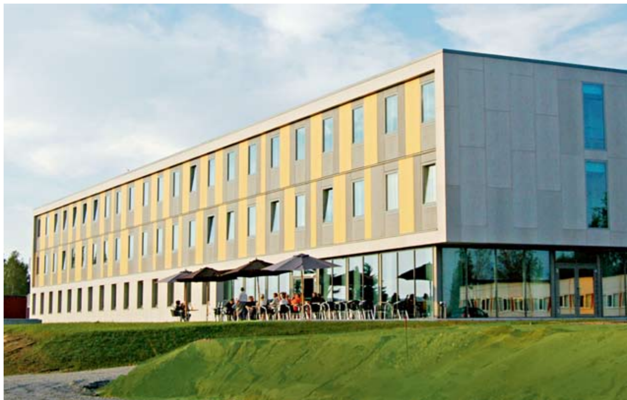
Moelven ByggModul AS has delivered 119 hotel room modules for Gardermoen Gjestegård. The overnight accommodation facility is located right next to the Oslo International Airport Gardermoen in Norway and opened in 2007. The hotel rooms are supplied complete with tiled bathrooms, installed bathroom fittings and heating and ventilation systems.
