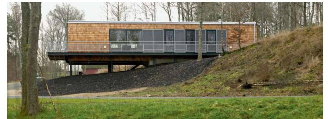
This Danish drawn, energy-efficient and environmentally certified (Svane) villa is located in Glimåkra, Skåne, in southern Sweden. The outside of the house is clad with Canadian cedar panelling supplied by Moelven Wood AB. The natural oils in the wood preserve the material so that the facade will not need maintenance for another 75 years.
