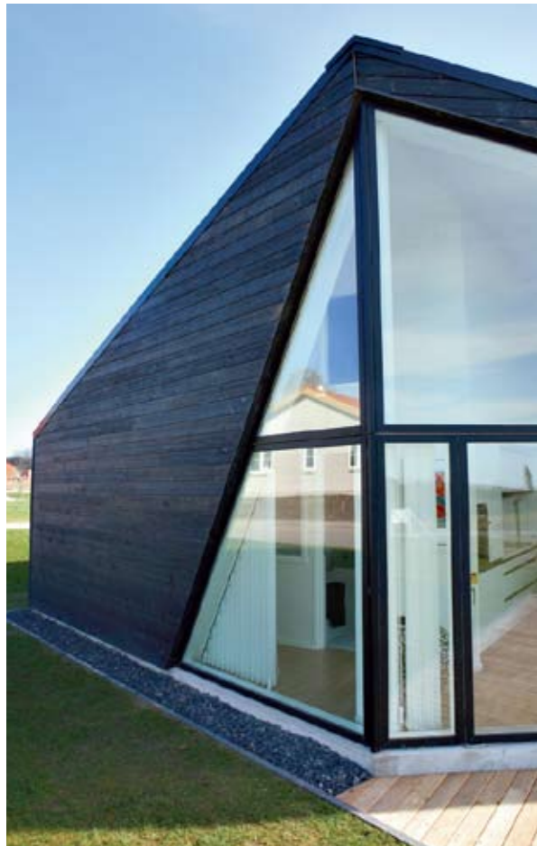
Wood supplied by Moelven Danmark AS has been used in visionary Danish house architecture. Kip House was drawn by the architectural firm 3XN and built by the construction firm M2. The wood used for the house was Finnforest ThermoWood, and had been heat-treated, base coated, finished and supplied ready for installation.
