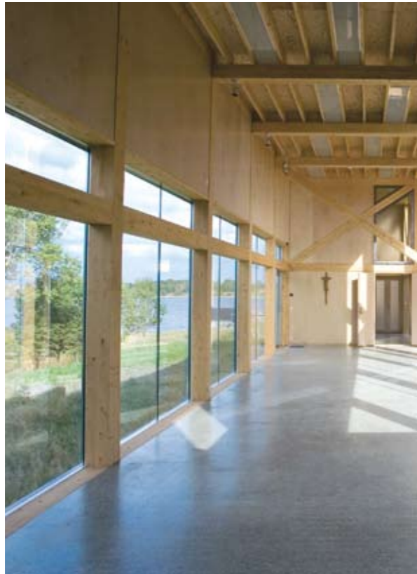
Large glulam beams for walls and roof were used to build the Tautra Maria convent located alongside the Trondheim fjord in Nord-Trøndelag in Norway. The laminated timber was supplied by Moelven Limtre AS. In 2006, the convent received the Building of the Year award in Norway.
