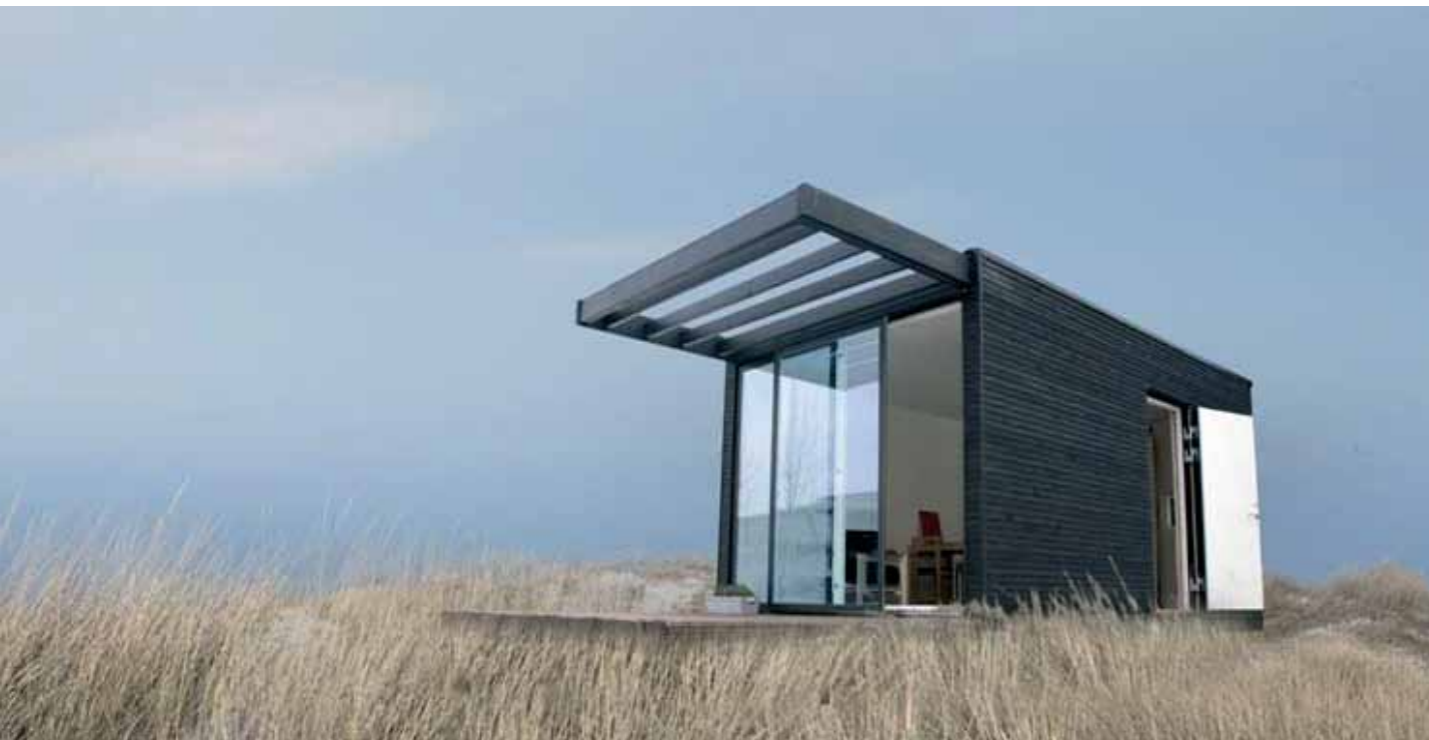
Minihuset ONE+, 15 m 2 , is built as prefabricated modules from organically-impregnated Swedish pine. Architect: Lars Frank Nielsen, manufacturer: Add-A-Room, Tyresö, Sweden.
