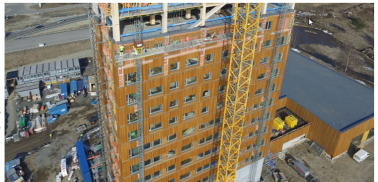
Figure 17 The timber structure was installed with the help of a tower crane as well as lifts positioned on the decks. No external scaffolding was used
