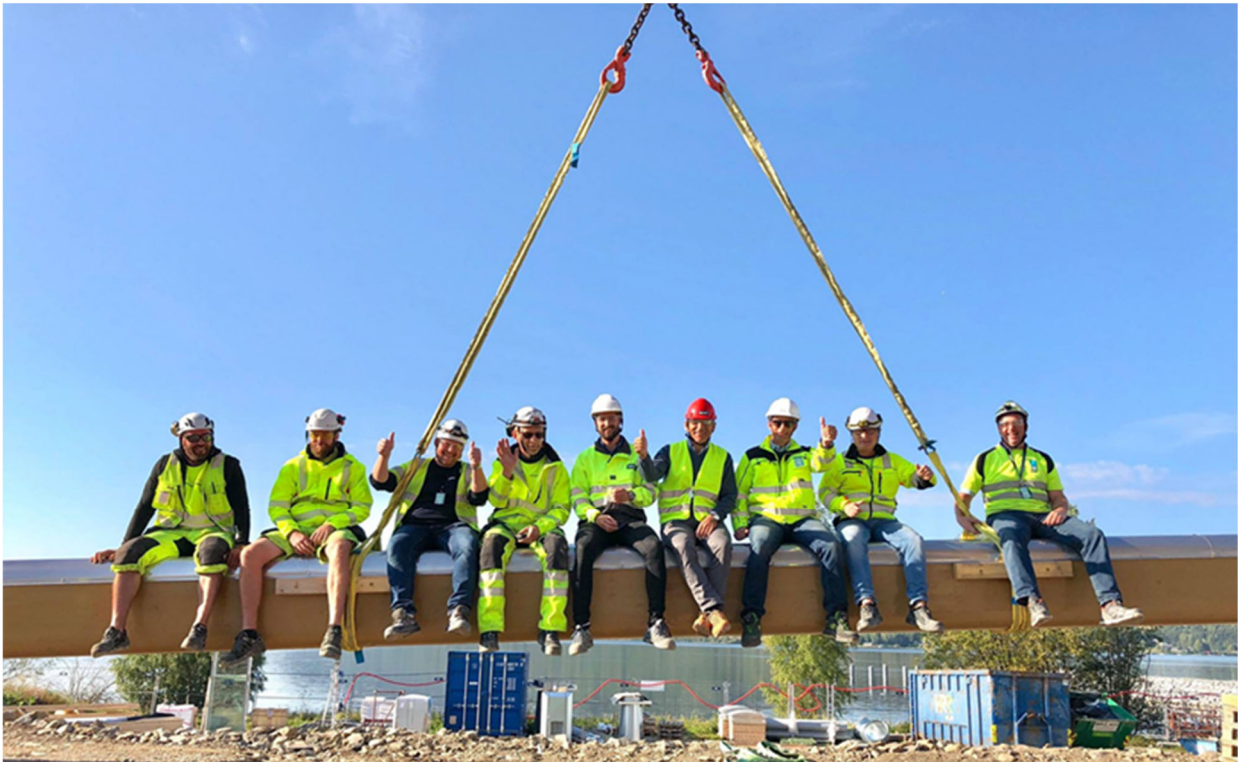
Figure 21 Image taken before the installation of the top beam on Sep 4, 2018
