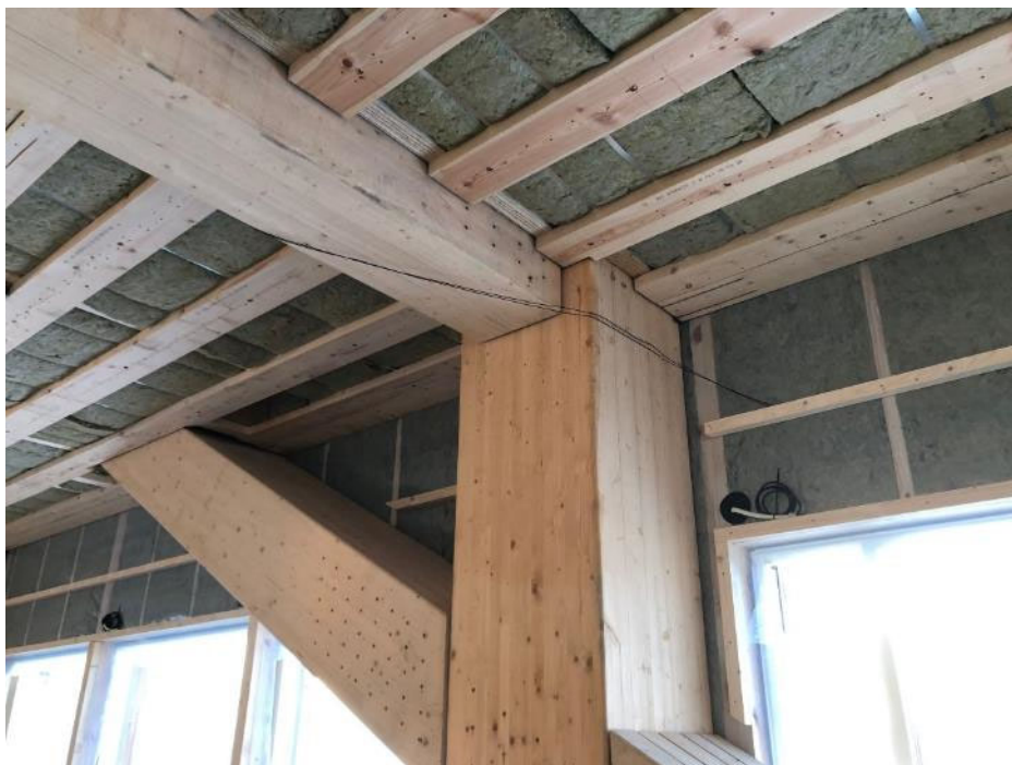
Figure 3 Accelerometers were installed directly onto structures
