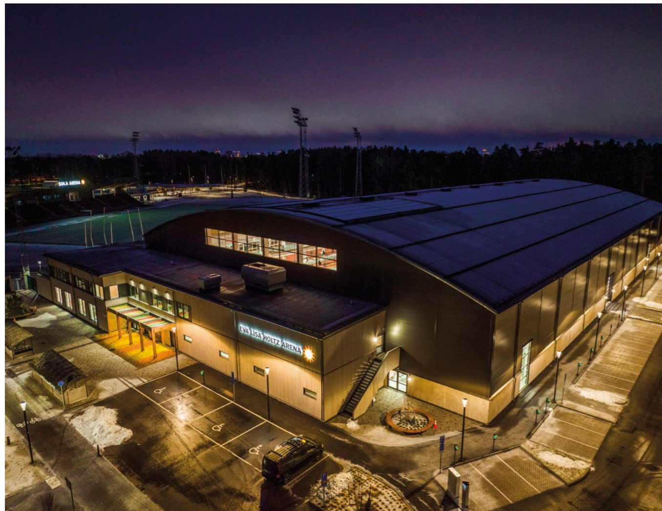
The brand new Eva Lisa Holtz Arena in Karlstad consists of several Moelven products. Moelven Töreboda AB has supplied glulam and cross laminated wood for the arena, while Moelven Wood AB is responsible for the external facade. Photo: Sören Håkanlind
