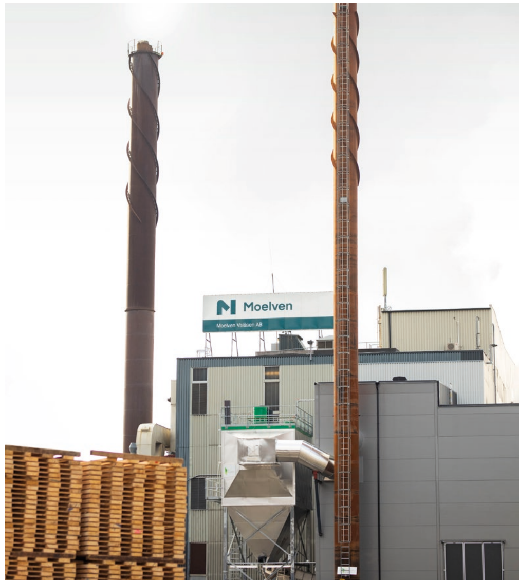
If you drive past Moelven Valåsen AB in Karlskoga today, you will be able to see smoke coming out of two chimneys instead of one like before. This is the result of the decision to invest MNOK 60, taken at the end of 2020. The new energy centre brings us one step closer in our efforts to make the sawmill more sustainable. At the same time, we have also ensured the operation of the new sawmill line, which is now being designed at Moelven Valåsen.
