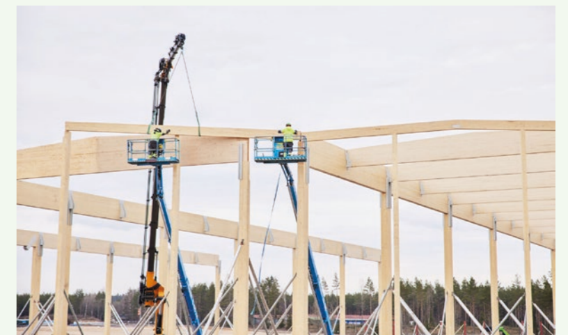
Elgiganten's new warehouse and logistics facility in Jönköping will be one of the largest in the Nordic region. Moelven's delivery consists of over 500 gable roof beams, and they are 24 meters long and almost two meters tall. The load bearing structure of the 86,000 square meter building consists entirely of glulam from Moelven Töreboda AB and Moelven Limtre AS. Photo: Sören Håkanlind and Jonas Ingman
